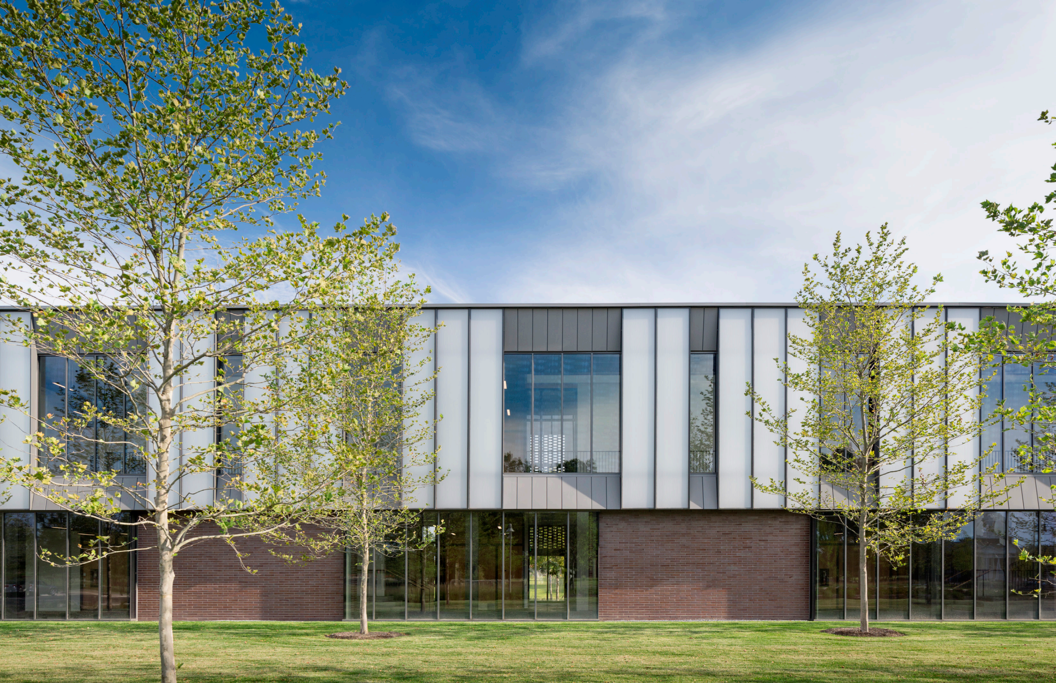
The north façade is comprised of 19-foot translucent panels that enhance the thermal performance of the exterior envelope.
